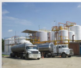
Bulk Liquid Receiving and Loading
